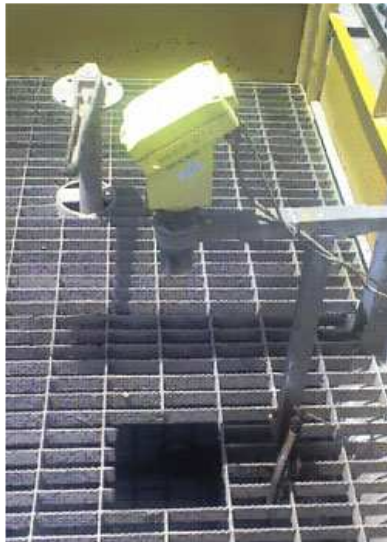
شکل 40 : Mud Level Recorder
